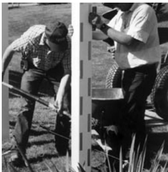
Post placement is important, using a stringline and level to assure vertical alignment.
